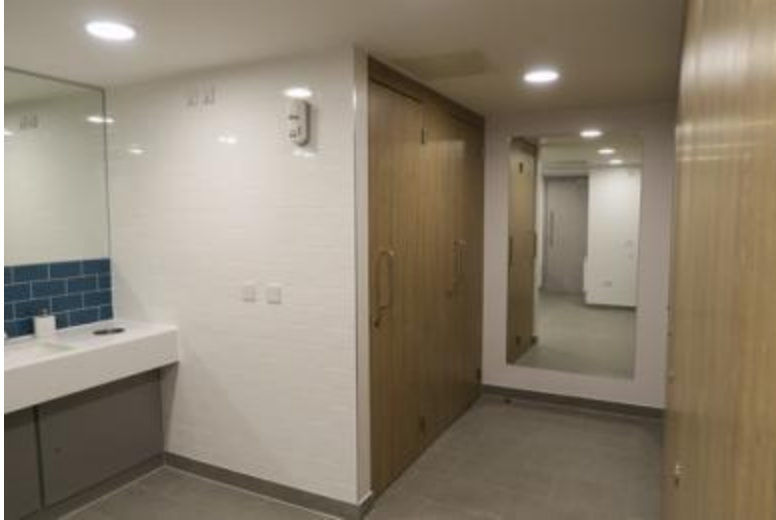
Outward opening doors in Aspects toilet facilities
