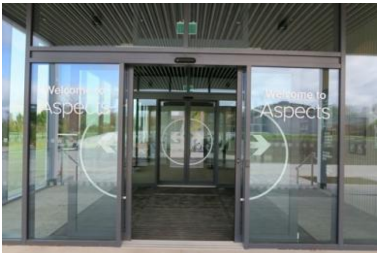
Aspects Building entrance lobby with 2 sets of automatic sliding doors
